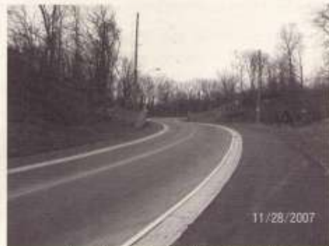
After the reconstruction the improvement is noticeable.
