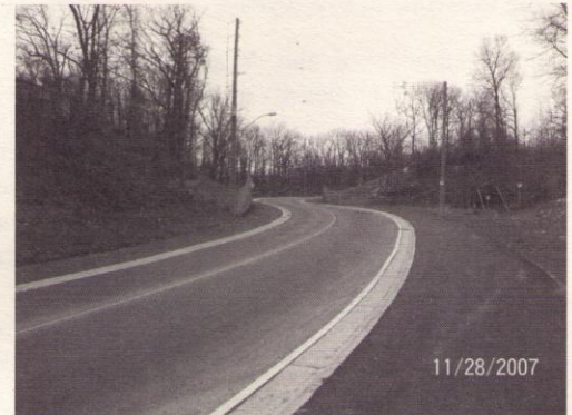
After the reconstruction the improvement is noticeable.
